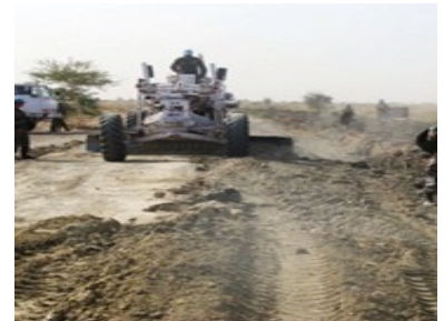
New roads to assist Malakal IDPs UNMISS Photo / Nyang Touch
