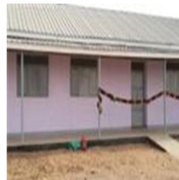
Two new classrooms for Warrap State UNMISS Photo/ Isaac Kelgbeh
